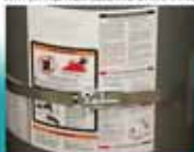
WATER HEATER SEISMIC STRAPPING
