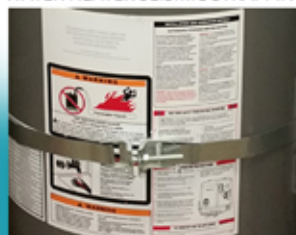
WATER HEATER SEISMIC STRAPPING
