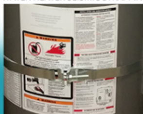
WATER HEATER SEISMIC STRAPPING
