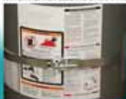
WATER HEATER SEISMIC STRAPPING
